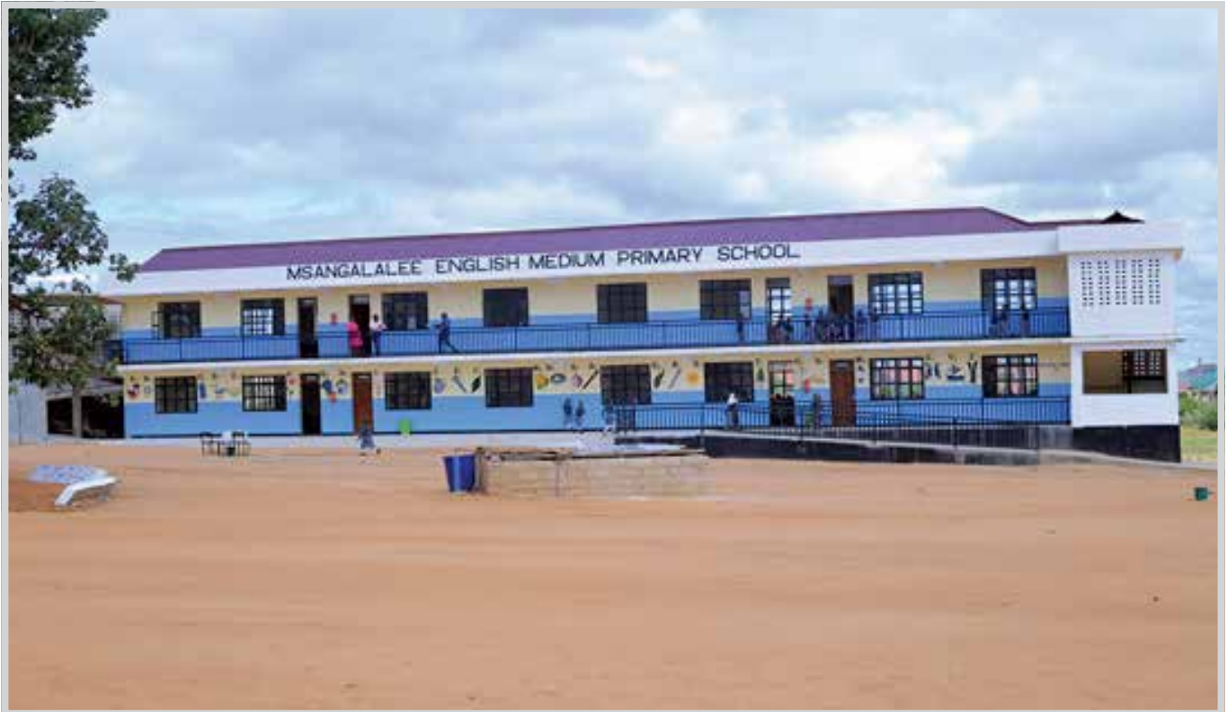
The view of Msangalalee English Medium School constructed with the support of the Education Fund in Dodoma.
