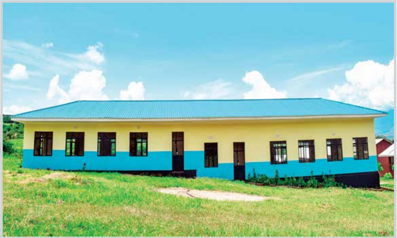
Chemistry and Biology Laboratory constructed under the Education Fund support at Maganjwa Secondary School, located in Babati DC Manyara region.
