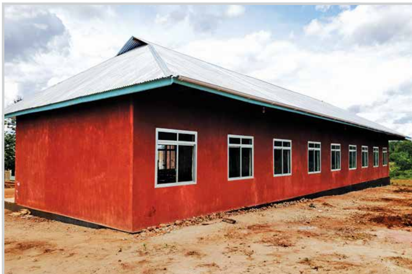
Three classrooms constructed at Kwaluguru Secondary School, located in the Handeni District of the Tanga Region.
