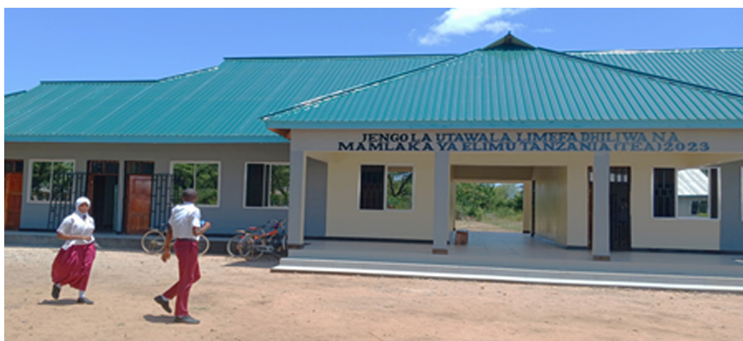
Figure 2: TEA funded administration Block for Ukenyenge Secondary of Kishapu DC in Shinyanga Region
