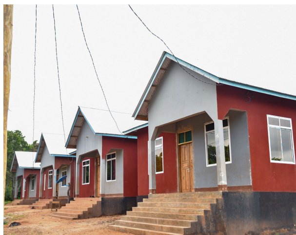
Four teachers' houses constructed by TEA at Mandarawe Secondary School, located in Ruangwa Municipality, Lindi Region.
